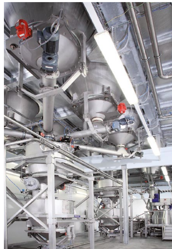
Exact dosing of the component batch sizes through dosing screws into the weighing bins. Pneumatic feeding into the dissolver-blender.
