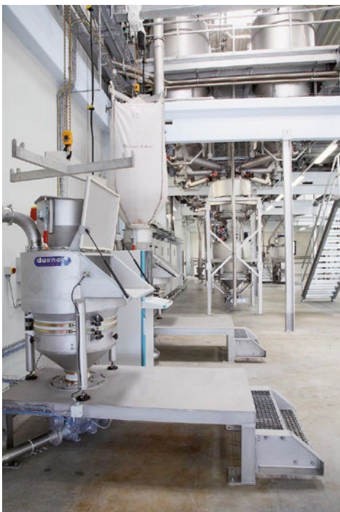
Loading station, where the product is fed out of bags and big bags; pneumatical conveying into the related day bin.
