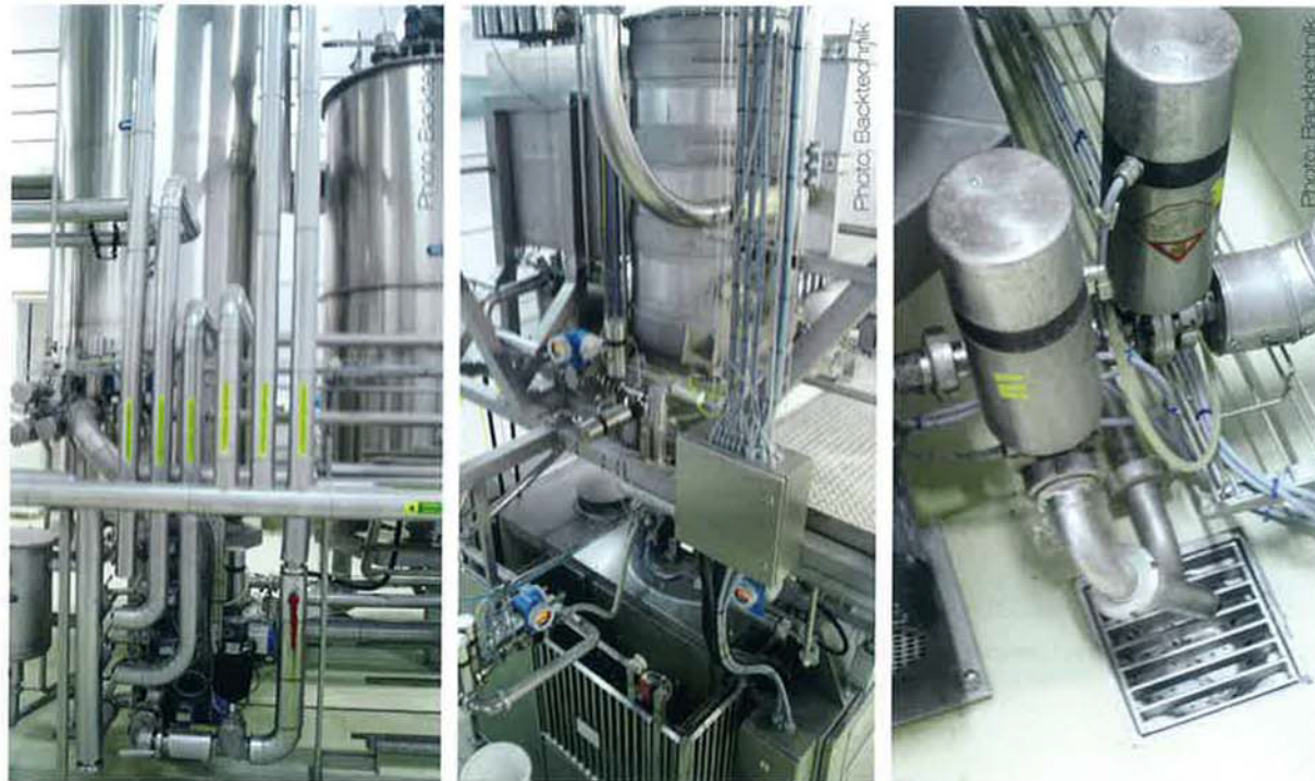
Left photo: An extensive cooling system ensures that the individual ingredients are at the desired temperatures. Middle photo: Daxner International has also delivered the plant system for weighing the product above the Turkington kneader. Right photo: The tanks can be emptied via the outlets on the diverse containers.
