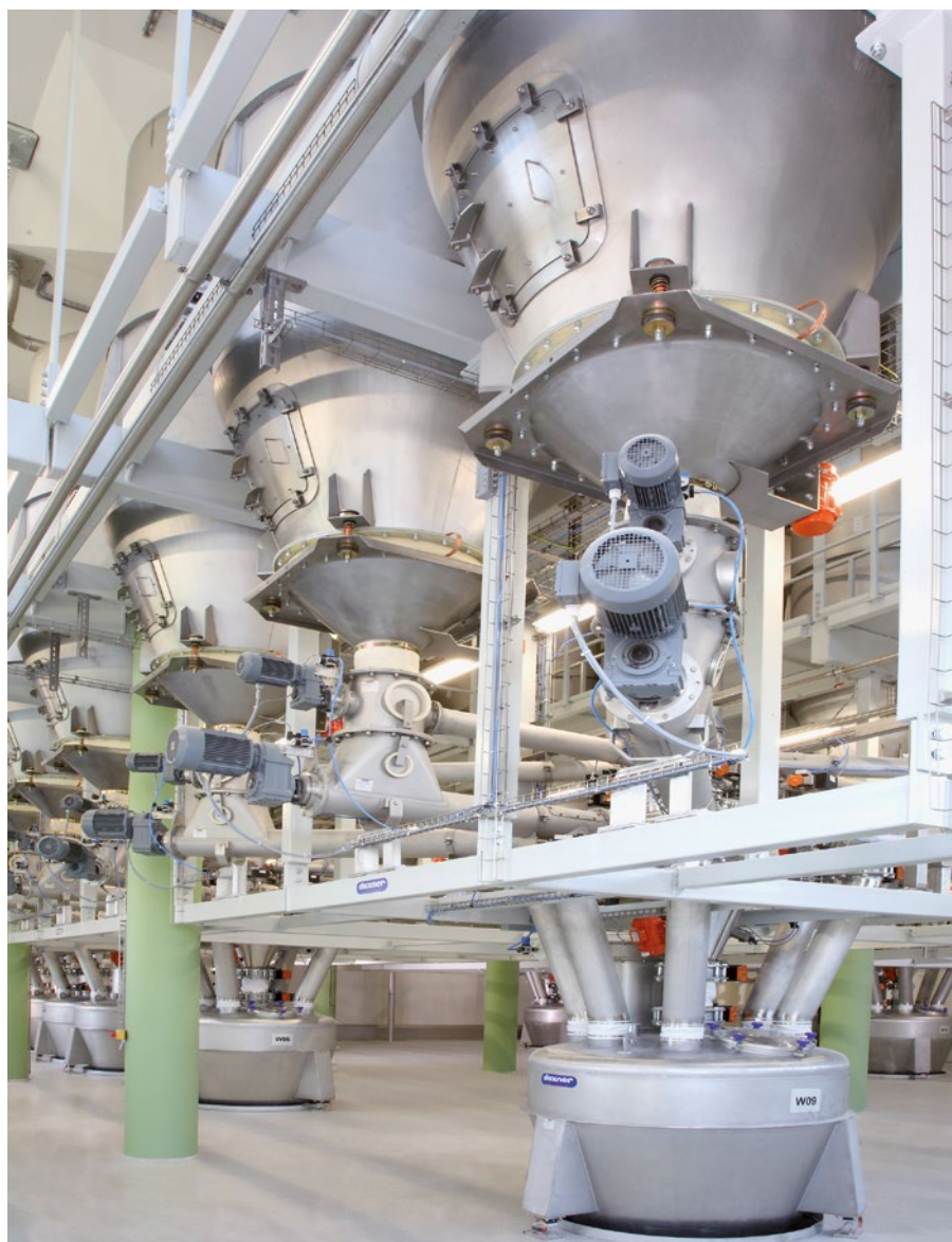
Dosing of raw materials with dosing screw and weighing vessel
