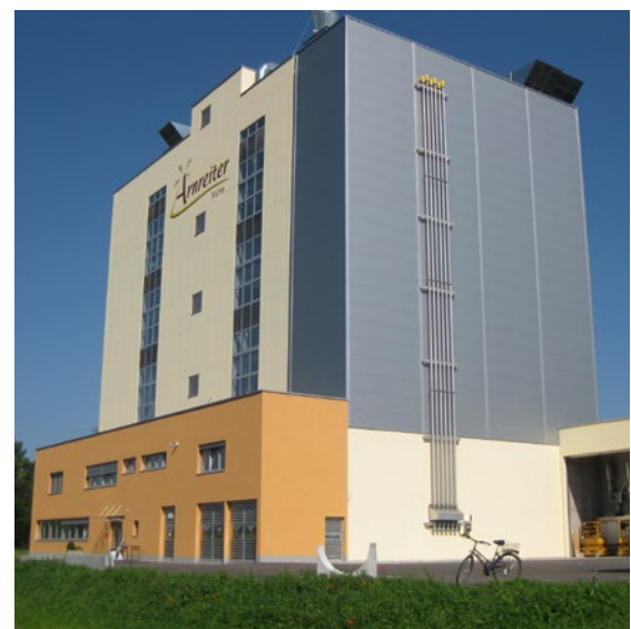
Outside view of building
