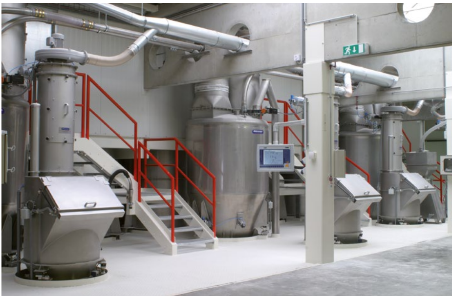
Bag intake system with control screens.
