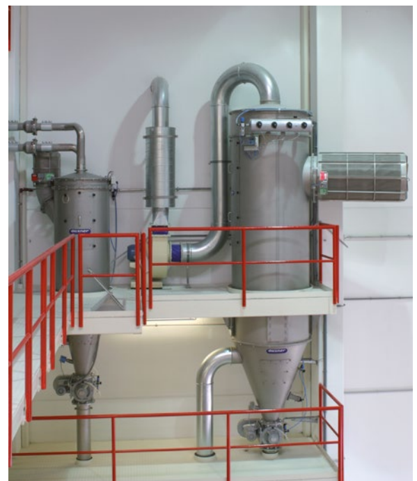
Central dust extraction system Explosion-proof design with Q-pipe, central aspiration with jet filter.
