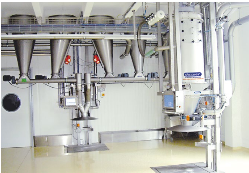
Automatic feeding and dosing of components into the dough shell
