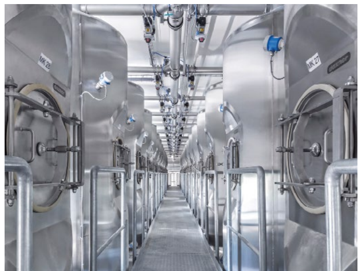
The middle components are stored in day bins and are loaded via a mobile Big bag discharge station.
