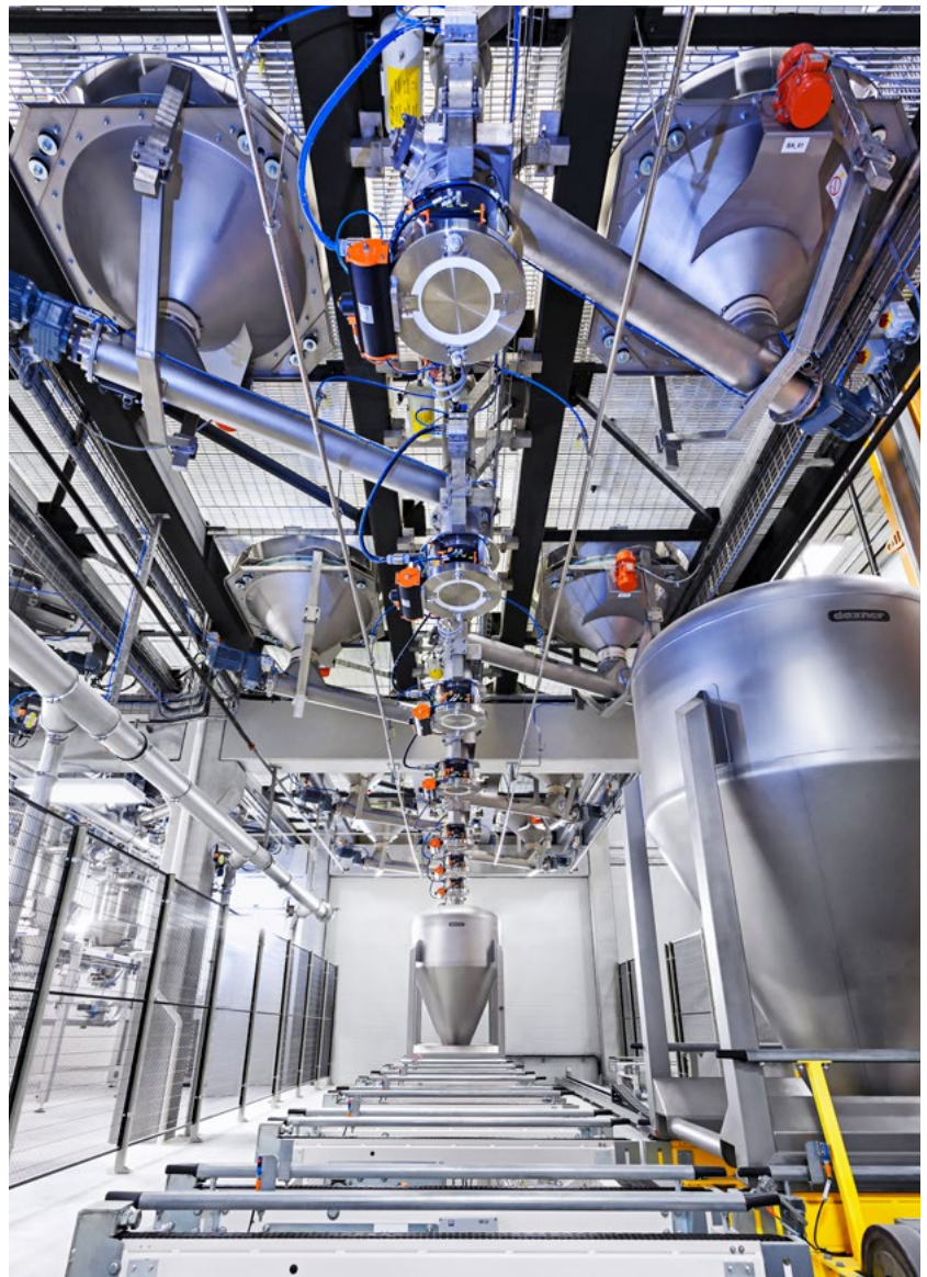
Fully automated ingredient handling system with Daxner Container Systems DCS.
