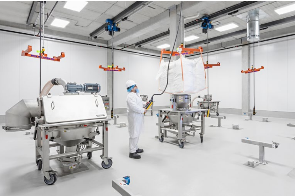
Mobile intake stations with integrated control screens for day silo loading of minor ingredients
