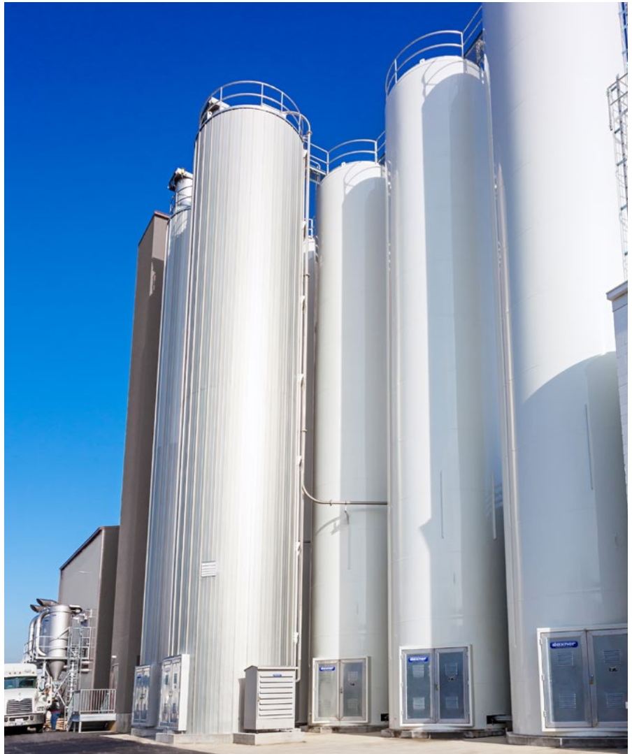
Outdoor silo system for major ingredients
