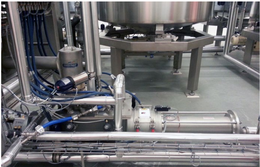
All tanks, both for sour dough and sponge, are mounted on load cells in order to precisely control the processing sequences. The pre-dough mixer mixes the individual components of the wheat sponge with a mixing screw to form a homogeneous mass.
