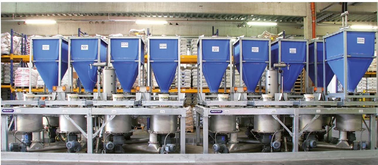
Batch component dosing facility System for 2 x 8 components Product infeed into standardized containers; Buffer bins with rotary bin dischargers; Dosing screw conveyors with flow stop discharge valve.
