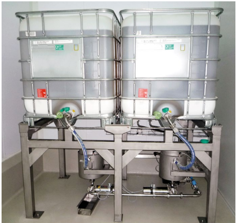
Two tanks provide for the sufficient oil quantity that is transported via a pump to the dough preparation unit and the kneader.
