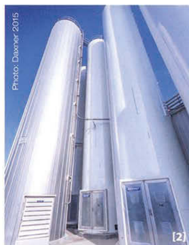
[1] Medium components are stored in day silos and filled by mobile feeding stations with integrated control screening machines. [2] Large components are stored in external silos and pneumatically fed to the mixing lines.
