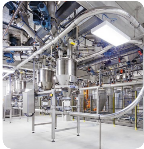
Pneumatic vacuum conveying system
