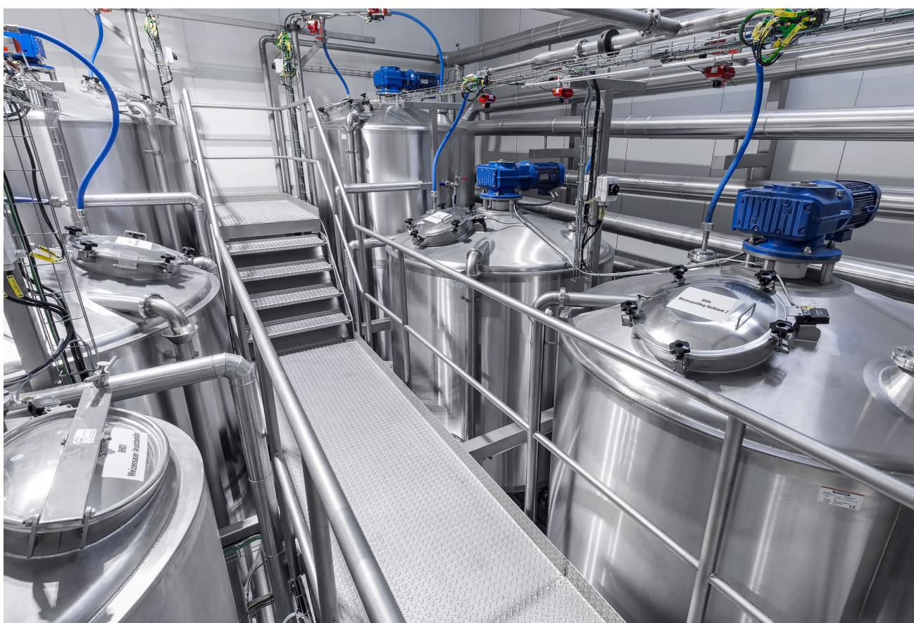
Storage tanks with mixer
