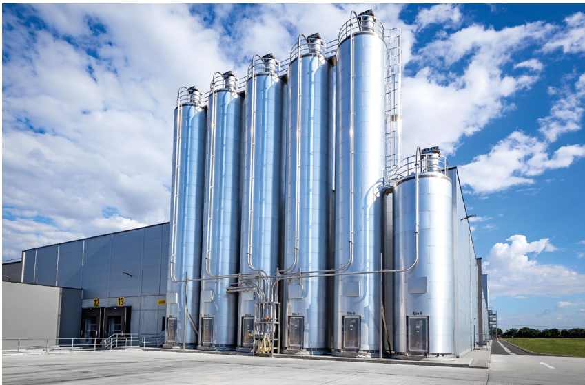
The six outdoor silos are filled pneumatically.
