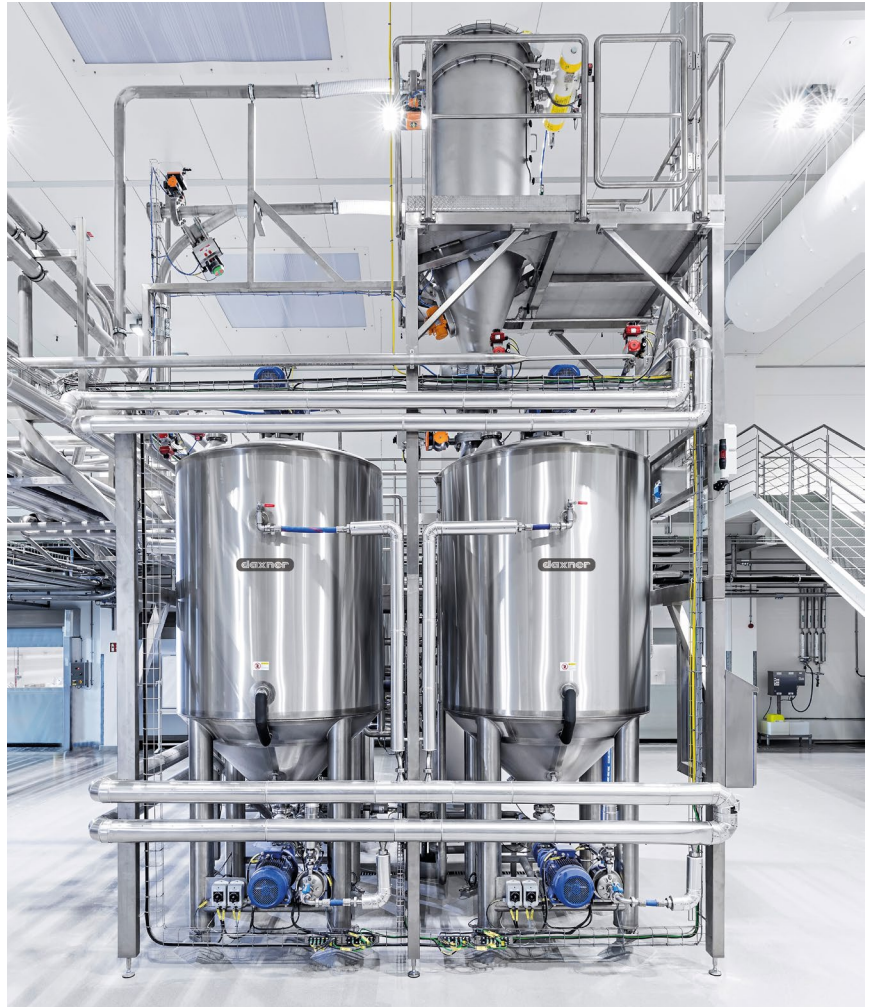
Soaking system with preparation and storage tank
