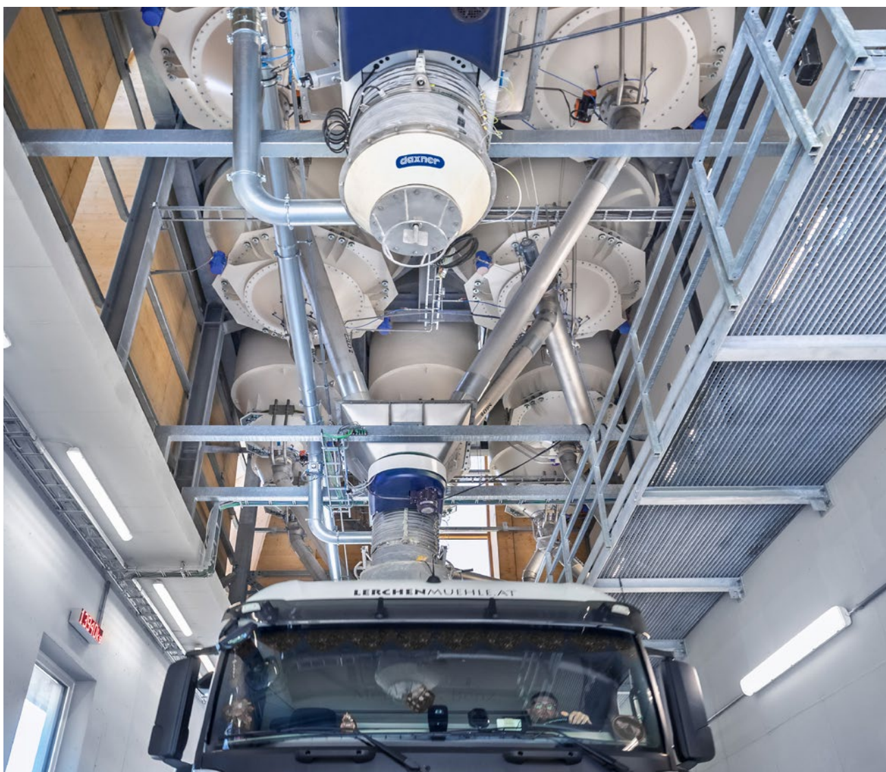
Dust-free truck loading in the protected loading hall
